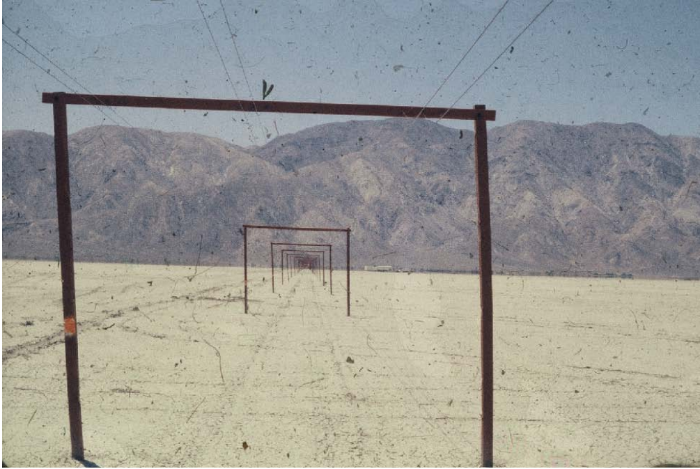
Figure 8. The open wire transmission lines carrying signals from the grating array.
