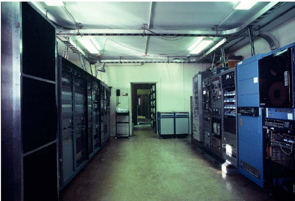
Figure 20. Receiver room with the analog receiving system and the correlator at left, solar equipment at right.
