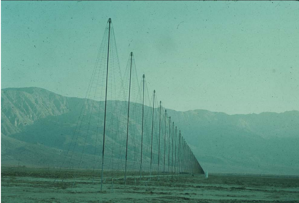
Figure 11. A view from the end of the south arm of the TPT.
