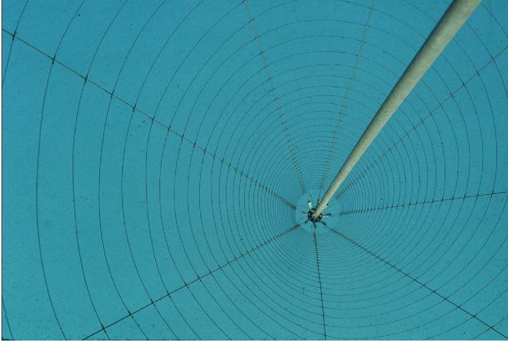
Figure 12. One of the TeePee elements. Eight ropes support the spiral wires that carry the RF signals.
