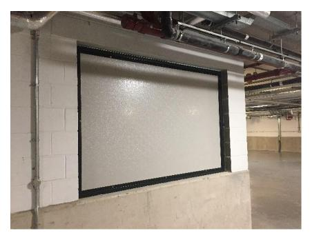
Intended to release overpressure from within buildings by allowing the panel to release from the frame.
