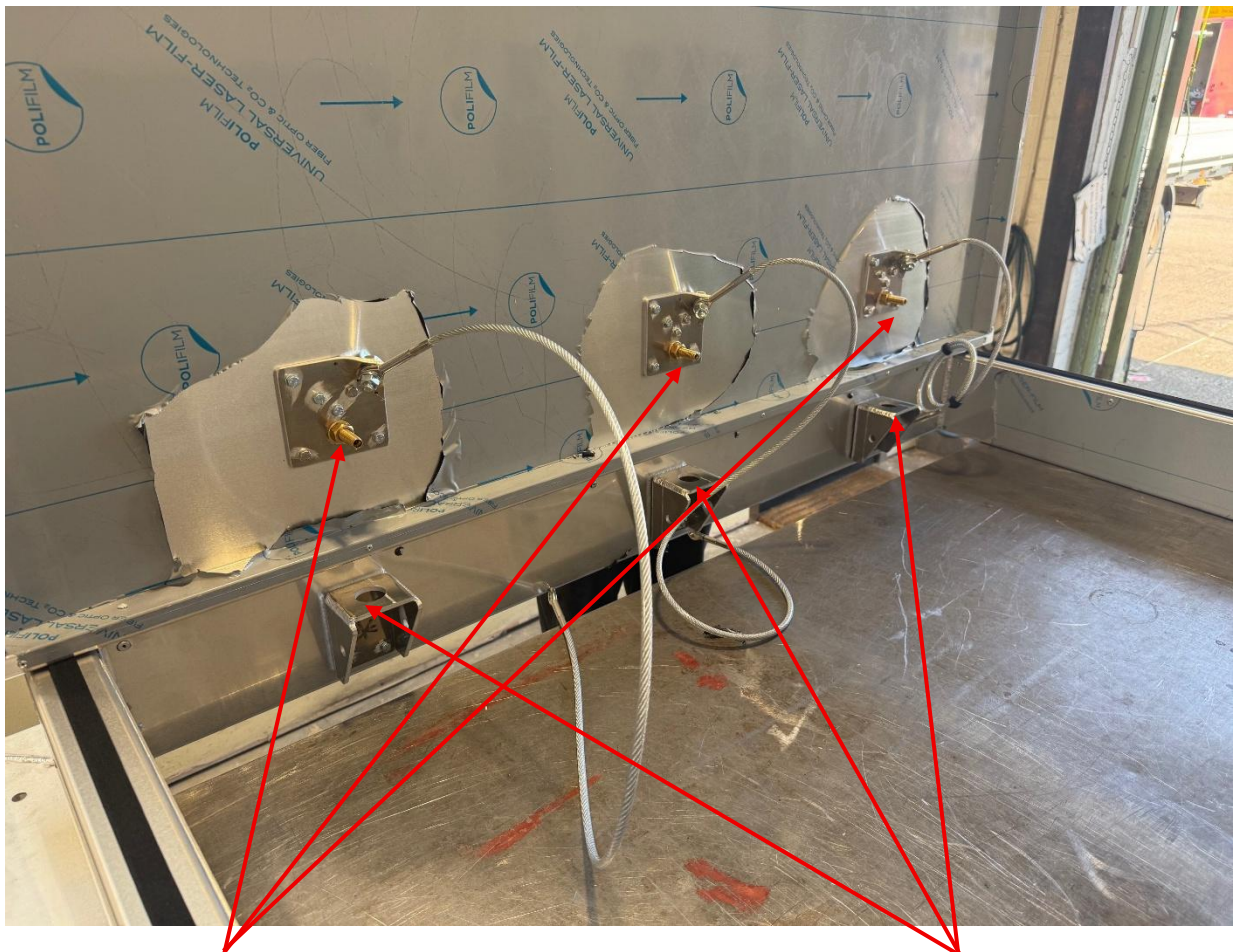
Connecting bolts on top panel of roof vent
