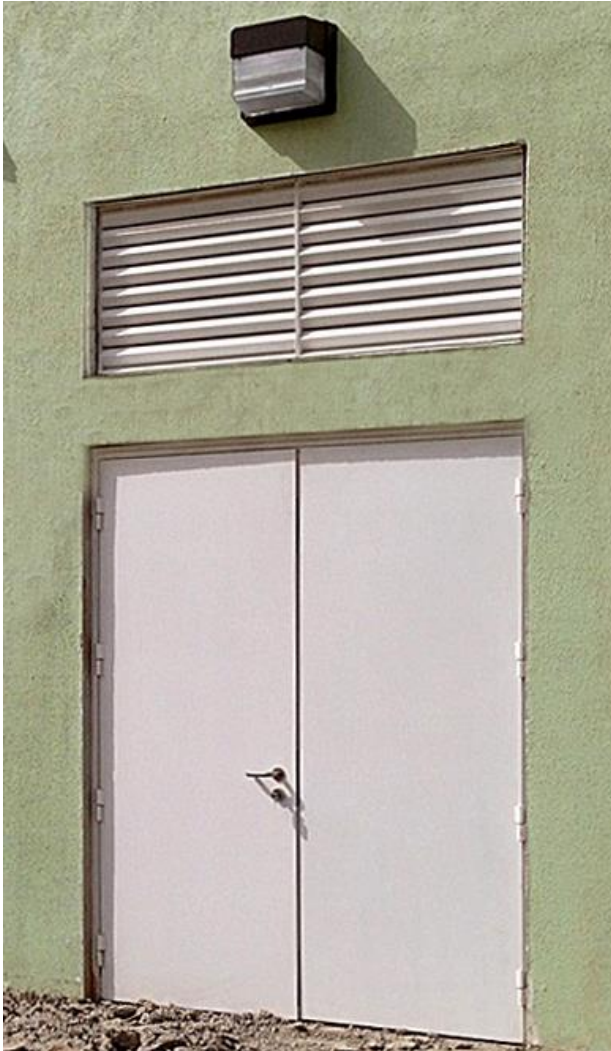
Double doorset installation with ballistic louver above
