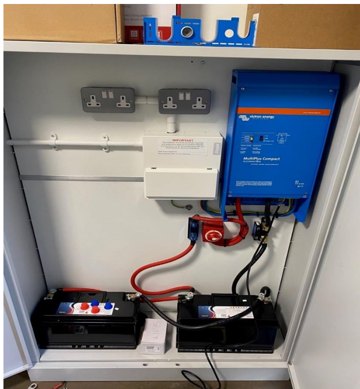
Emergency power back up including Lithium Battery
