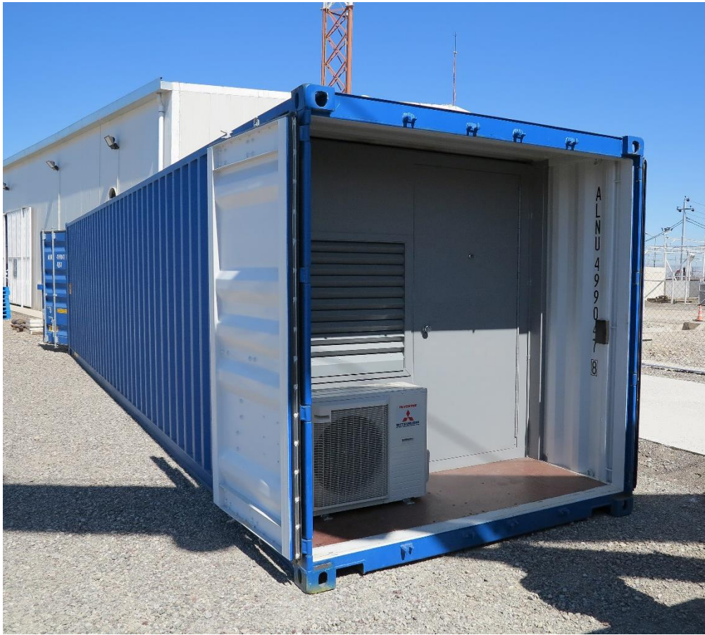
Inner lobby area with ballistic louvers and door, also containing air conditioning and other plant and equipment
