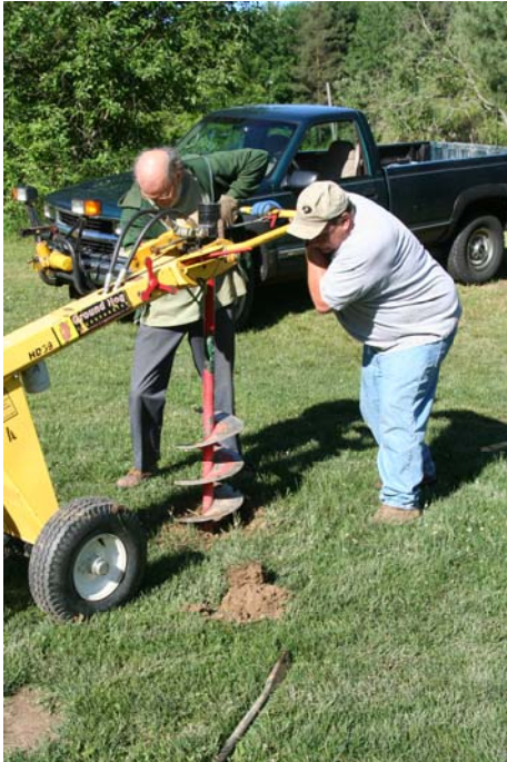
Left: Marty and Dan Rothstein drilling more holes for the piers that will support the roll-off roof.
