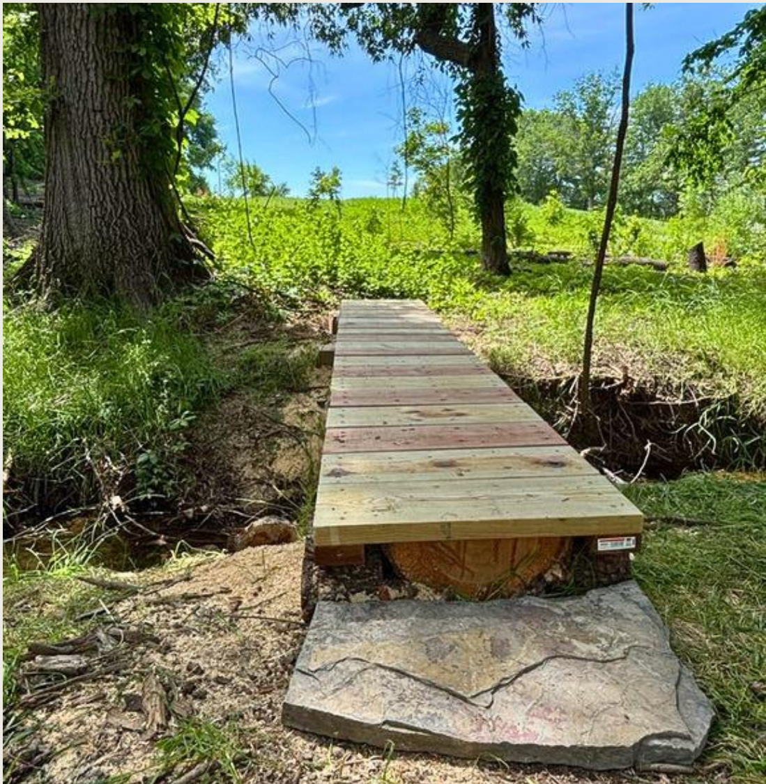
Warson Park New Pedestrian Bridge
