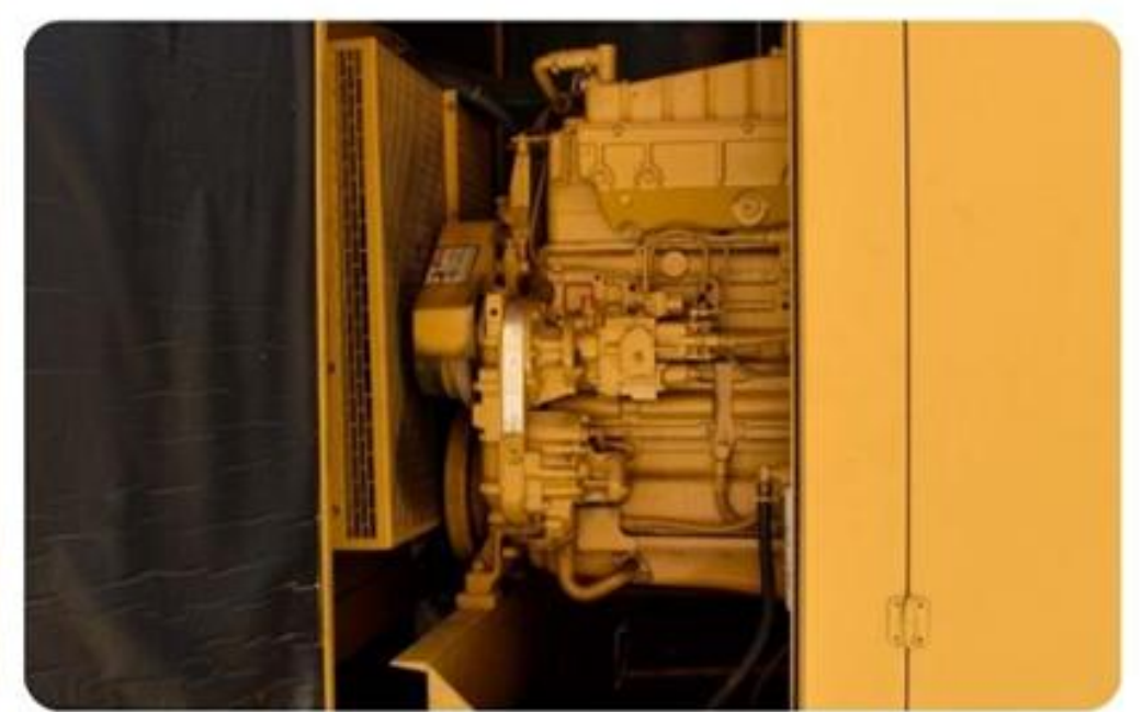
Aging Building Systems
