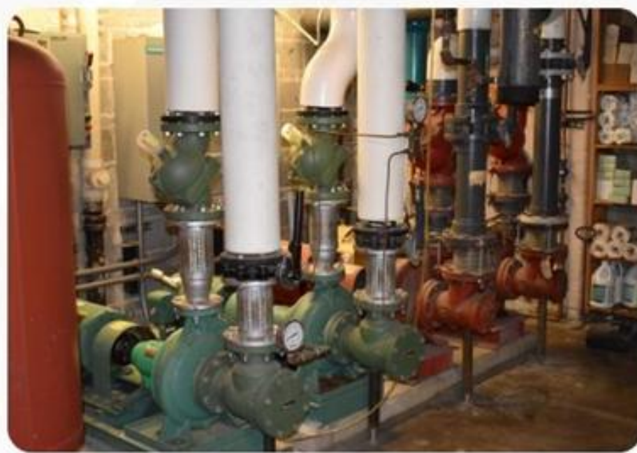
Aging Building Systems
