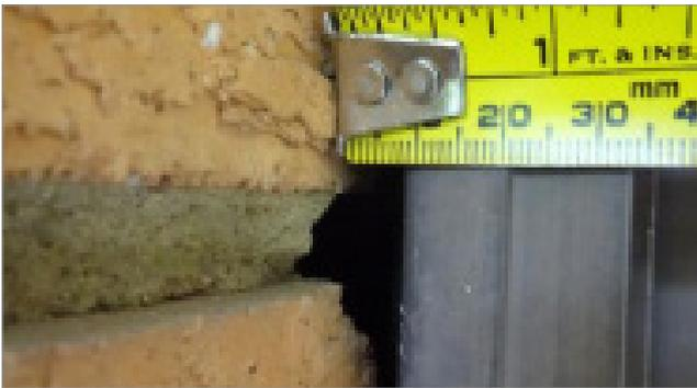
**Figure 9** A gap on the external wall surface between frame and brickwork.
