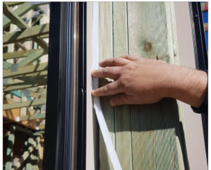
**Figure 12** Applying high density acoustic foam to the exterior of the window frame.
