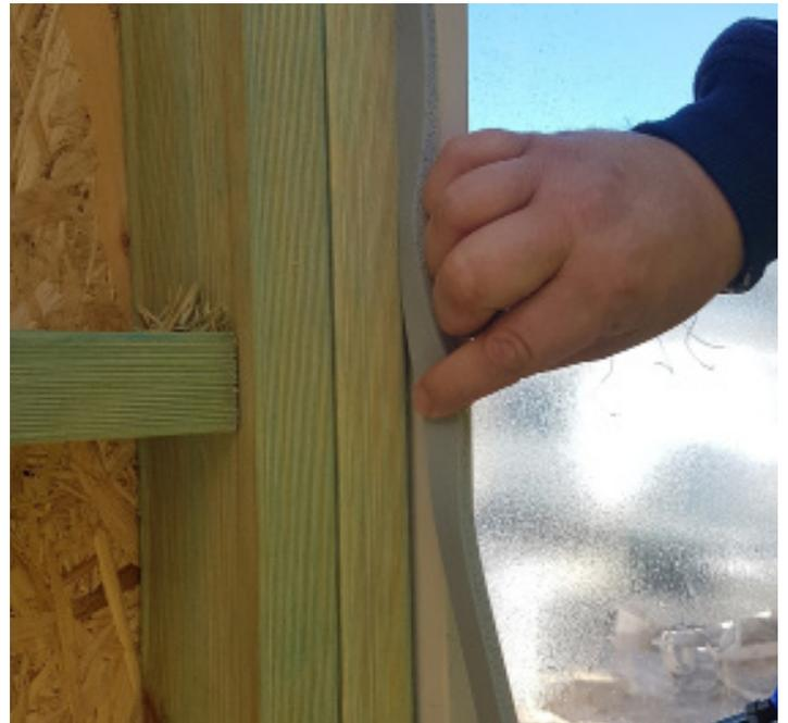
**Figure 11** Applying high density acoustic foam
