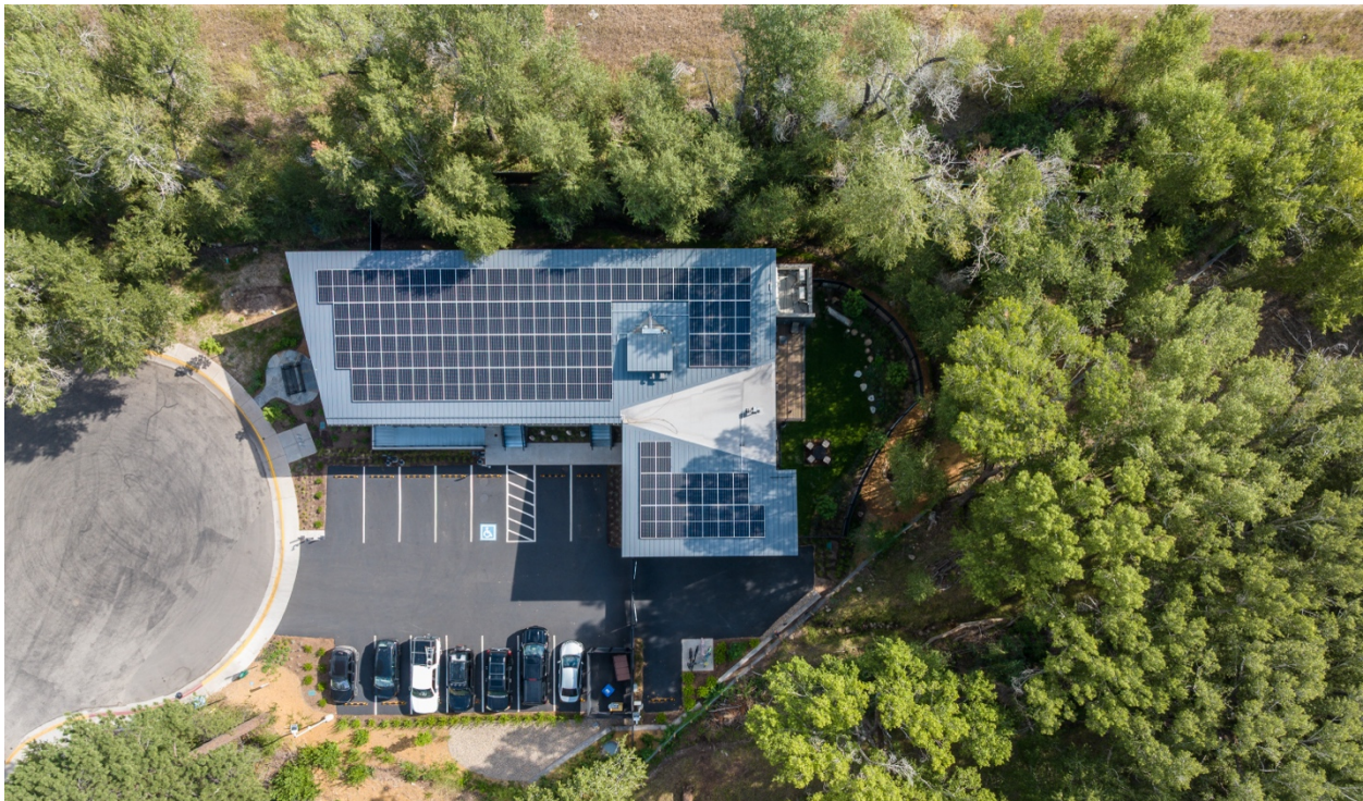
View of solar panels on the roof of Halle Center for Hope and Healing
