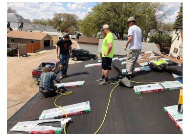
Fixing the rectory roof
