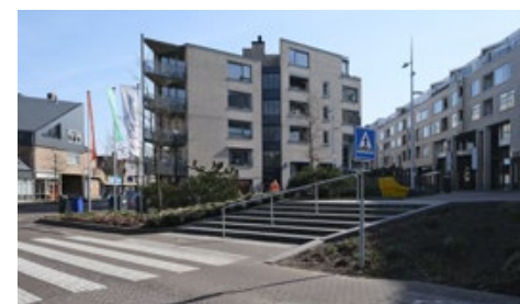
Overgang Markt - Emmaplein
