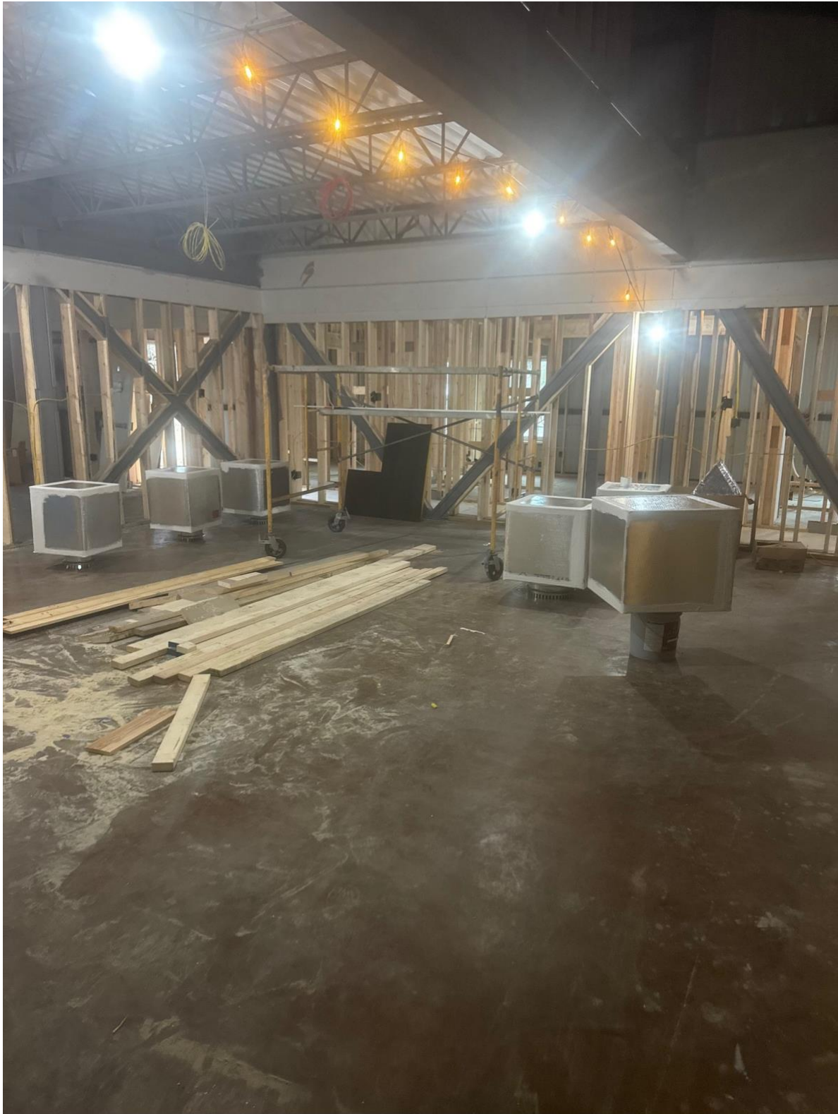
Interior view of the station, showing wiring in progress, plenums for HVAC
