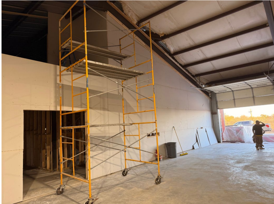
Photo 7 – One Hour Firewall being installed between Apparatus Bays and Dayroom / Offices
