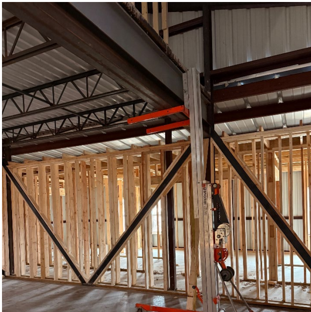
Photo 2 - Structural reinforcement of specified beams and columns
