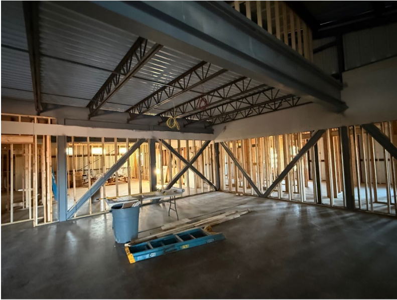
Photo 3 - Structural reinforcement of specified beams and columns
