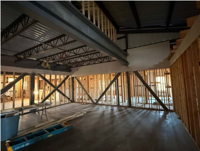
Photo 4 - Structural reinforcement of specified beams and columns
