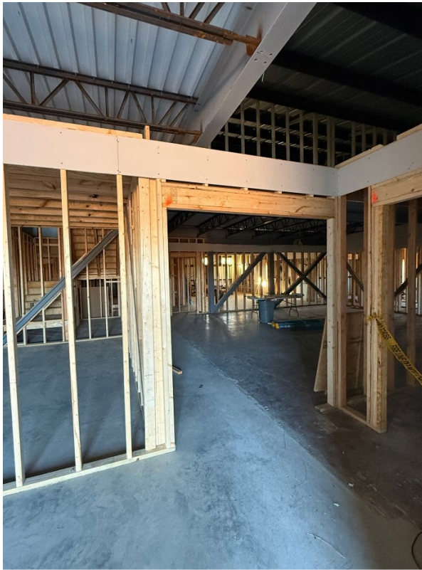
Photo 6 – Example of Completed Framing
