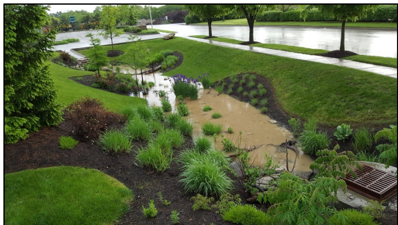
Figure 2: A typical stormwater bioswale that combines natural filtration with an underground media filter. Image courtesy of the Klaus Group.
