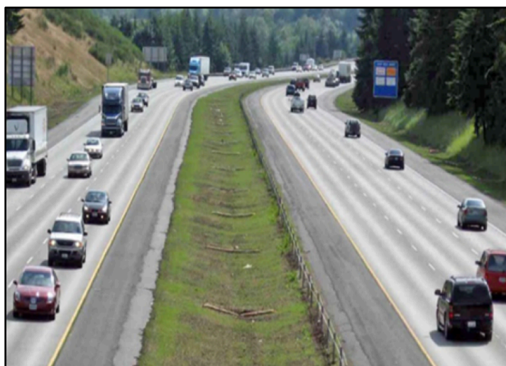
Figure 10: Compost amended vegetated filter strips are beginning to be deployed along the interstate highway system to treat metals and sediments. They also hold promise for 6PPD-Q reduction (WSDOT, 2023).
