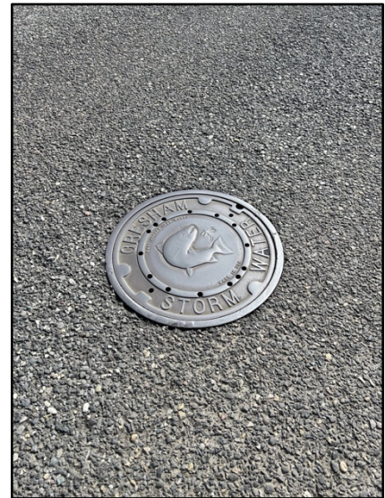
Figure 4: Porous asphalt overlay in Gresham, Oregon, 17 years after installation.
