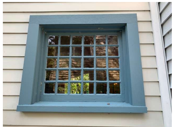
21. Original window reused in new addition
