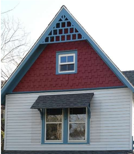
15. Hooded window and stickwork on west gable end
