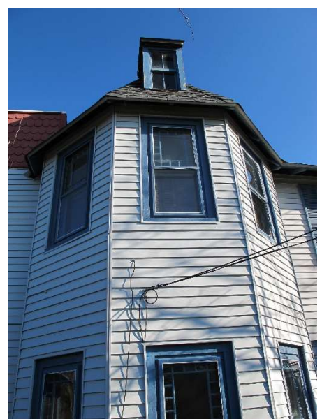
14. Two story bay
