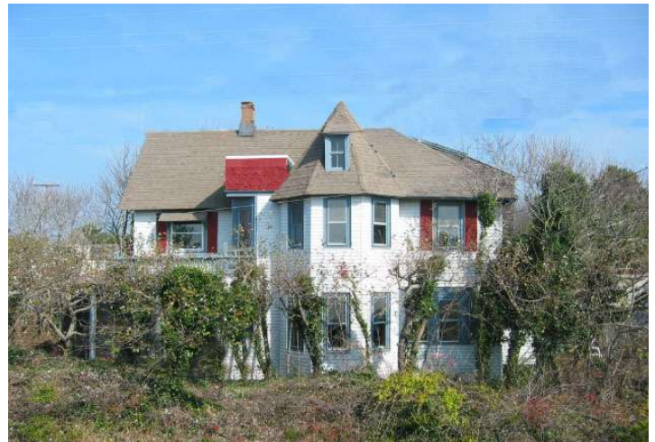
45. 2008 prior to 2010 renovation
