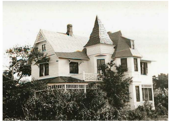
41. 1930's photo showing exterior details before tower roof was destroyed
