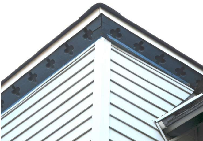
20. North tower quatrefoil motif at soffit bargeboard
