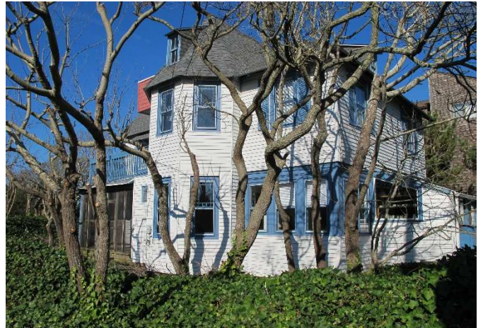
4. View from driveway (southeast)
