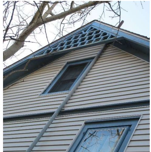
16. Stick work at north gable
