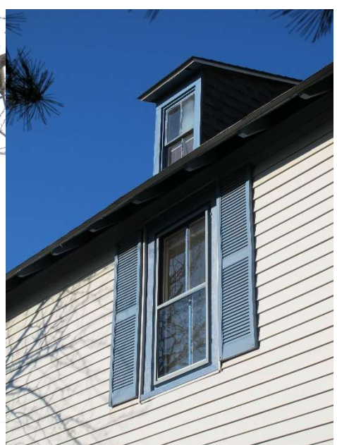
19. 2 over 2 sash east facade
