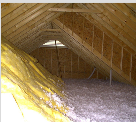
Blown and Batt insulation in attic.
