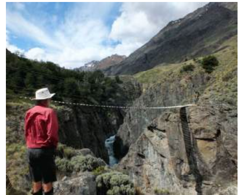
Parque Patagonia bridge
