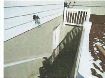
Walk up Basement Exit
