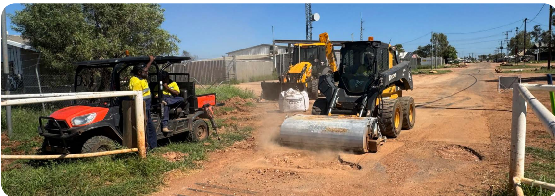
Work at Football Oval in Alpururulam
