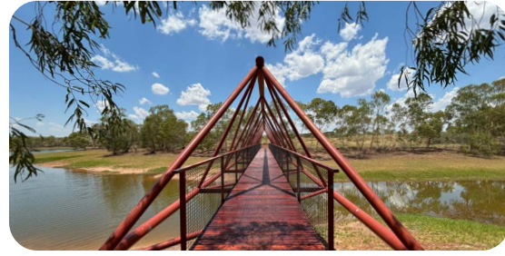
Lake Mary Ann (Tingkarli) Walk Bridge Upgrade
