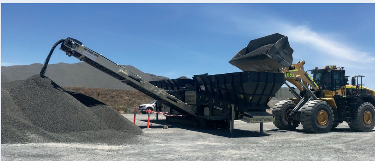
Blenders - Pugmills - Concrete Plant Silos
